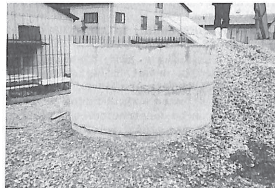
Plate 7 Foundation of electric supply frame constructed in the reinforced zone immediately behind the rigid facing during construction
